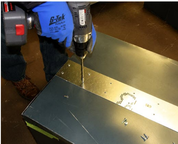
Figure 8. Fasten sheet metal over cut seam
